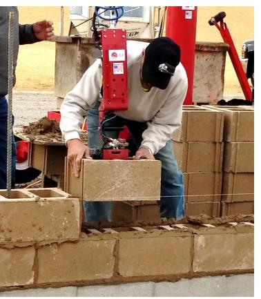
Specially designed griper works with most common brick sizes and types
