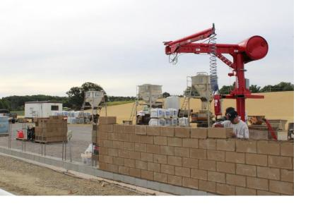
Ergonomic handling of masonry blocks reduces wear and tear on the masons body
