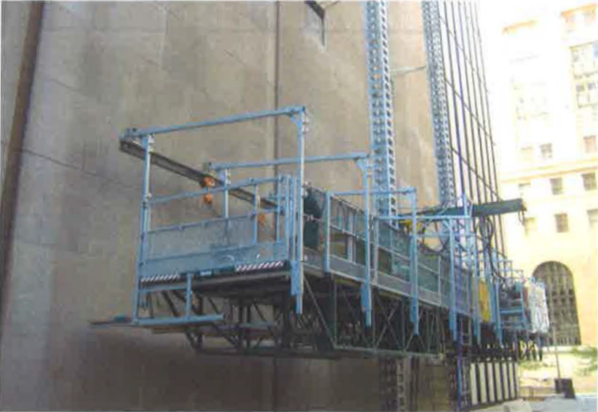
Photo 9: Mast Climber with Non-Swinging Mounted Monorail Hoist
