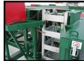
Open deck design to pass wall ties. New climbable tower w / quick connect bolts, no X-braces
